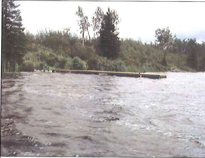
PHOTO 37 Fixed dock within Cabin6 Area.
