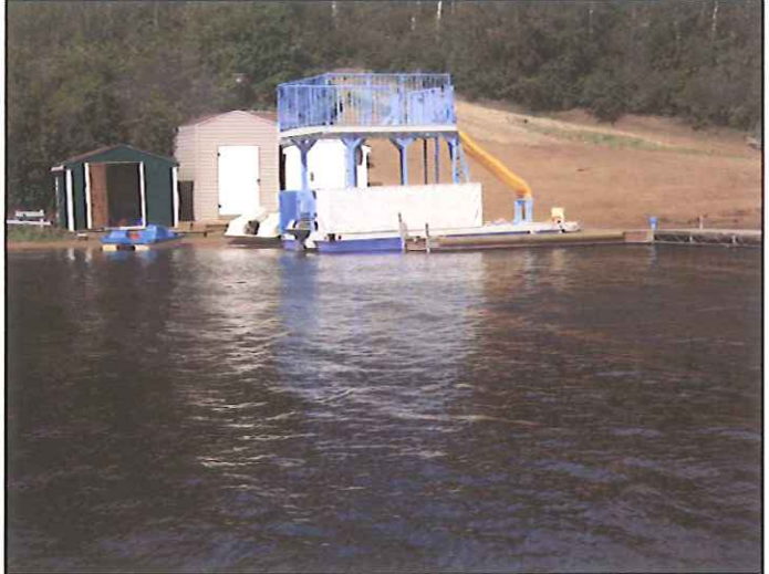
PHOTO 2 Dock and barge at Cabin1.
