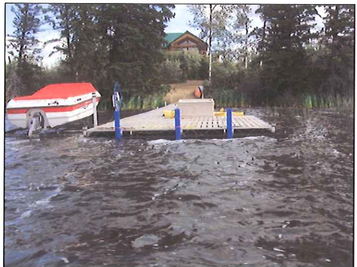
PHOTO 36 Fixed dock within Cabin6 Area.
